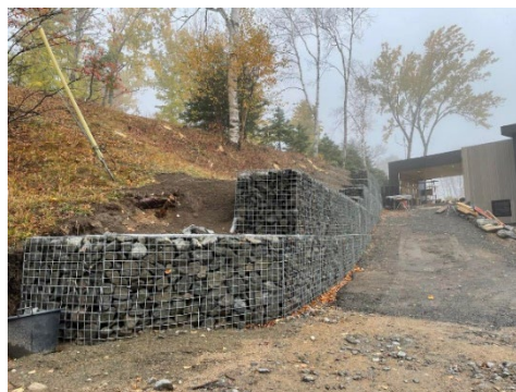
Le Gabion Structural
